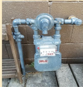
Decking built around piping and Fixture against meter
