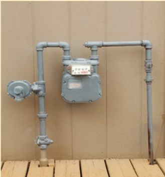
Decking built around service
