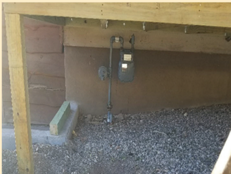
Deck built over an existing meter
